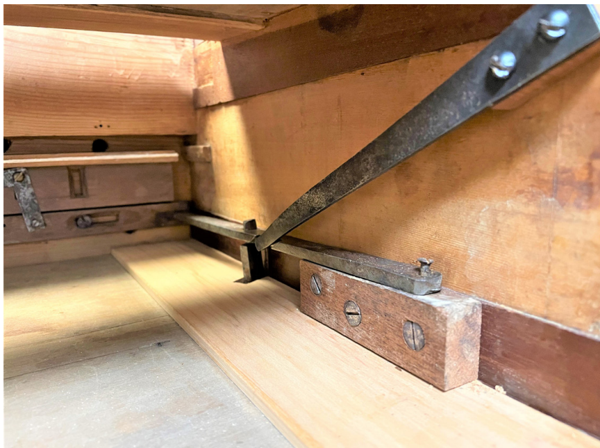
FIGURE 9. The damper-raising mechanism.
