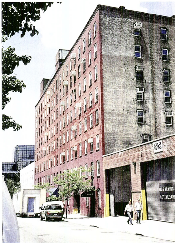
FIGURE 6. Joseph P. Hale's Factory no. 5, south elevation. Photograph by the author, 2007.
