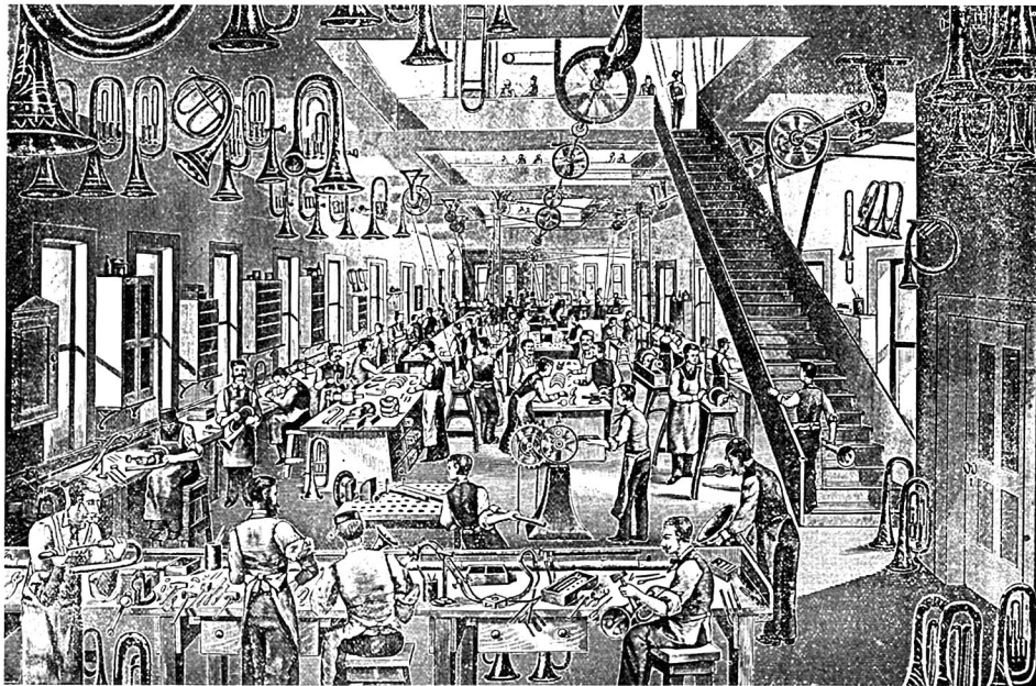
FIGURE 10. The horn-making department in the Conn factory, ca. 1894. Woodcut by Joe K. French. Courtesy of Lillian and Stuart Caplin.
